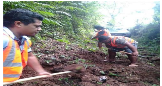
Landslide clearing works for access to Alaoa West WL Station
