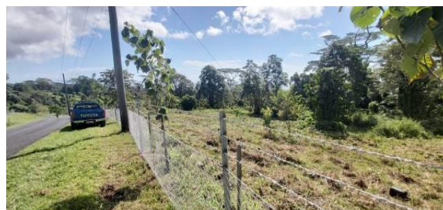
Methodist land rehabilitation works
