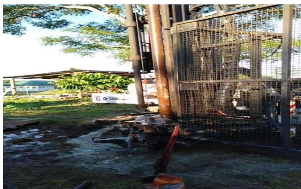
Drilling works at Vaipouli
