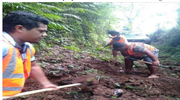
Landslide clearing works for access to Alaoa West WL Station
