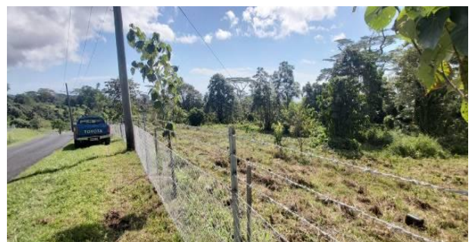
Methodist land rehabilitation works
