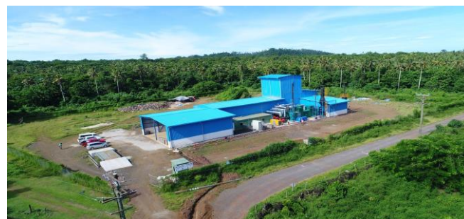
Afolau Biogas Plant
