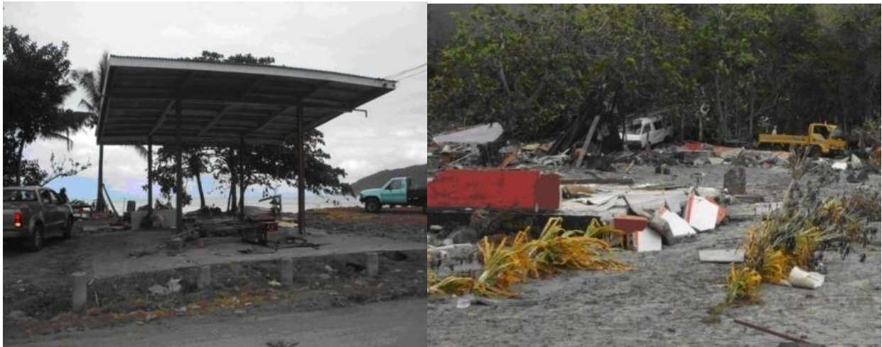
Figure 9 Retail store damage in Malaela and Petrol station in Vailoa
